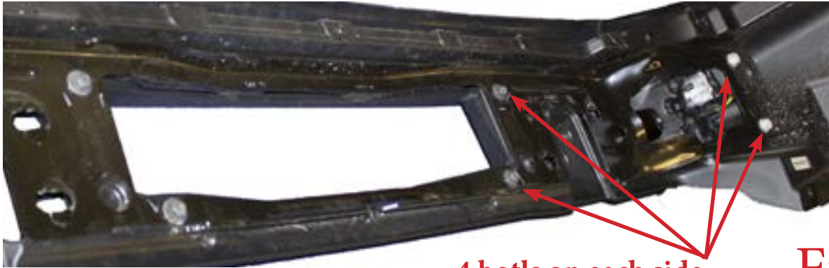
4 bolts on each side
