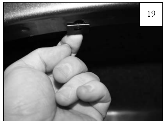
Install Clip (CL1-0022) over existing hole.
