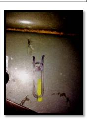
**Step 6:** Remove clip. Use a ½" drill bit and drill out the center mark. Slide the 3/8 clip back into position so the threaded part is aligned with the hole.
